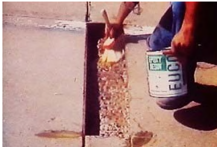
Figure 8. Application of Bonding Agent
