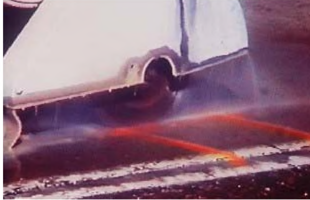
Figure 3. Diamond -bladed saw for Sawing & Chipping
