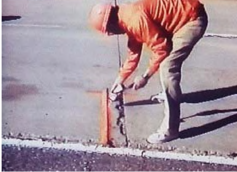
Figure 2. Marking Area for Removal
