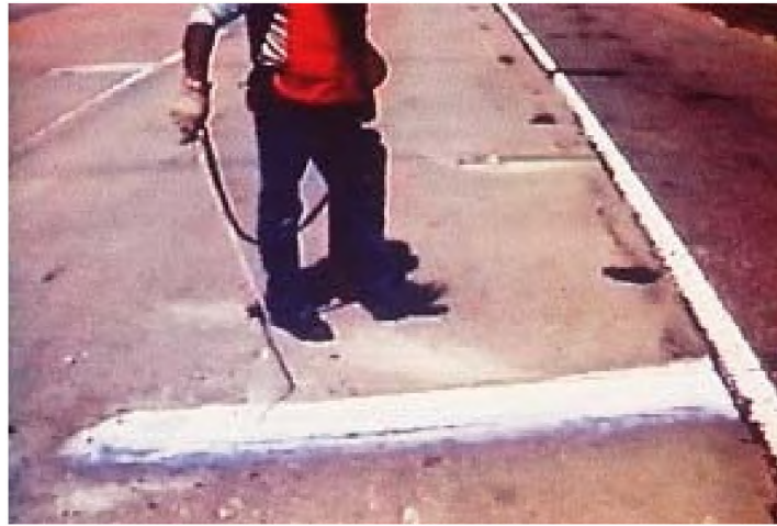
Figure 9. Application of Curing Compound
