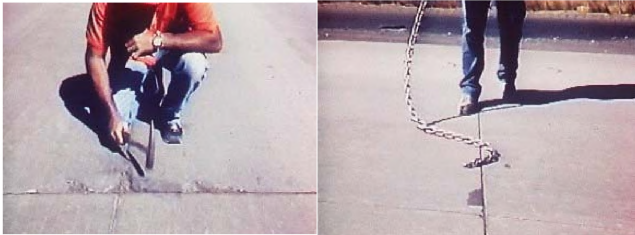
Figure 1. "Sounding" with ball-peen hammer (left) and steel chain (right)
